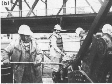
Fig. 1. Collection of the Buffalo River sediment. (a) The derrick boat and clamshell bucket used to collect the sediment. (b) The transfer of sediment with a Teflon-coated shovel from the clamshell bucket to a plastic-lined steel drum.
